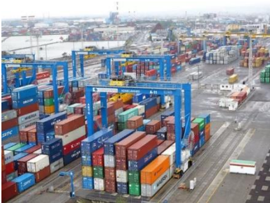
Figure 3(a). Rubber Tyred Gantry (RTG) (Konecranes, 2023b).
