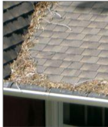
Figure 26. Debris accumulation behind a gutter cover. Photo: Stephen L. Quarles.
