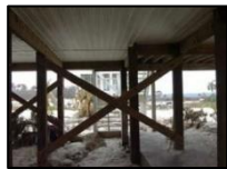
Figure 40. Open foundation (FEMA, 2008a).
