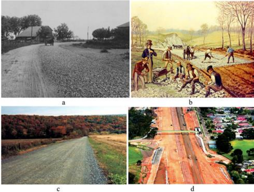
Figure 1: Development of earth roads. a, b Examples of "Macadam Roads", c: crushed stone road bonded with gravel, d: roller compacted earth road. (Lay, 2009, Anonymous 2023).
