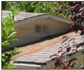
Figure 17. Needles (debris) from nearby pine trees have accumulated on the lower roof section (Division of Agriculture and Natural Resources).
